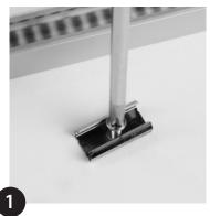
Fix clips with suitable screws (min. 2 per metre/40"). Mark & drill holes if required.
